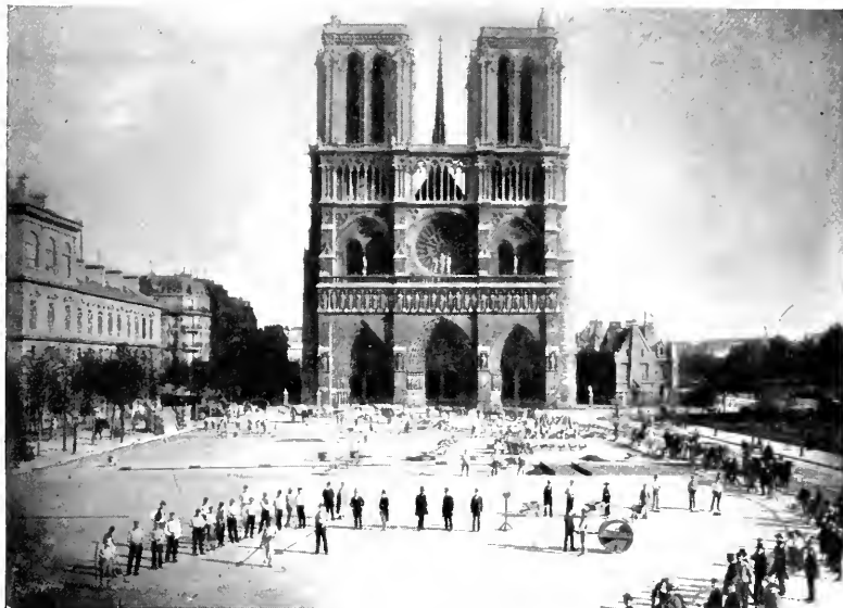
PARIS. ESPLANADE BEFORE NOTRE DAME CATHEDRAL. Laying asphalt pavement for vehicles, foot traffic, processions, and ceremonies.
